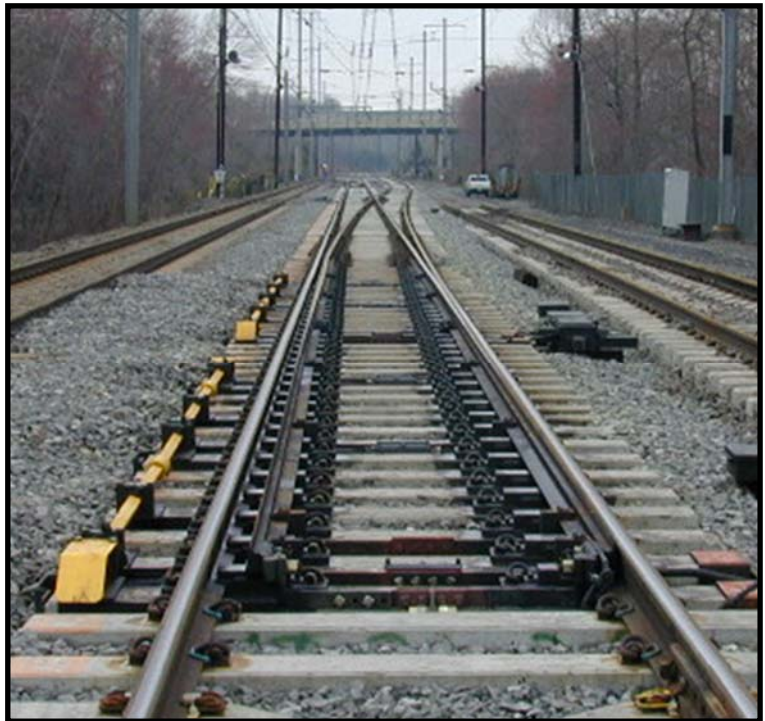
M-3 Switch Machine (High Speed)
