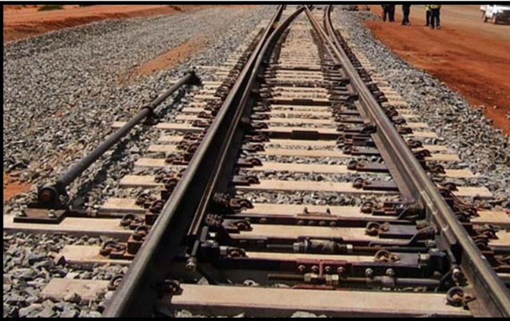
Rotary Helper Rod Layout
